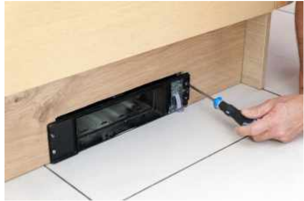
21. Screw into place using the 4 wood screws.
